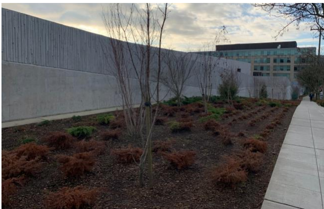
Figure 3 - This photo is of the outside of the Wallingford-Fremont transfer station
